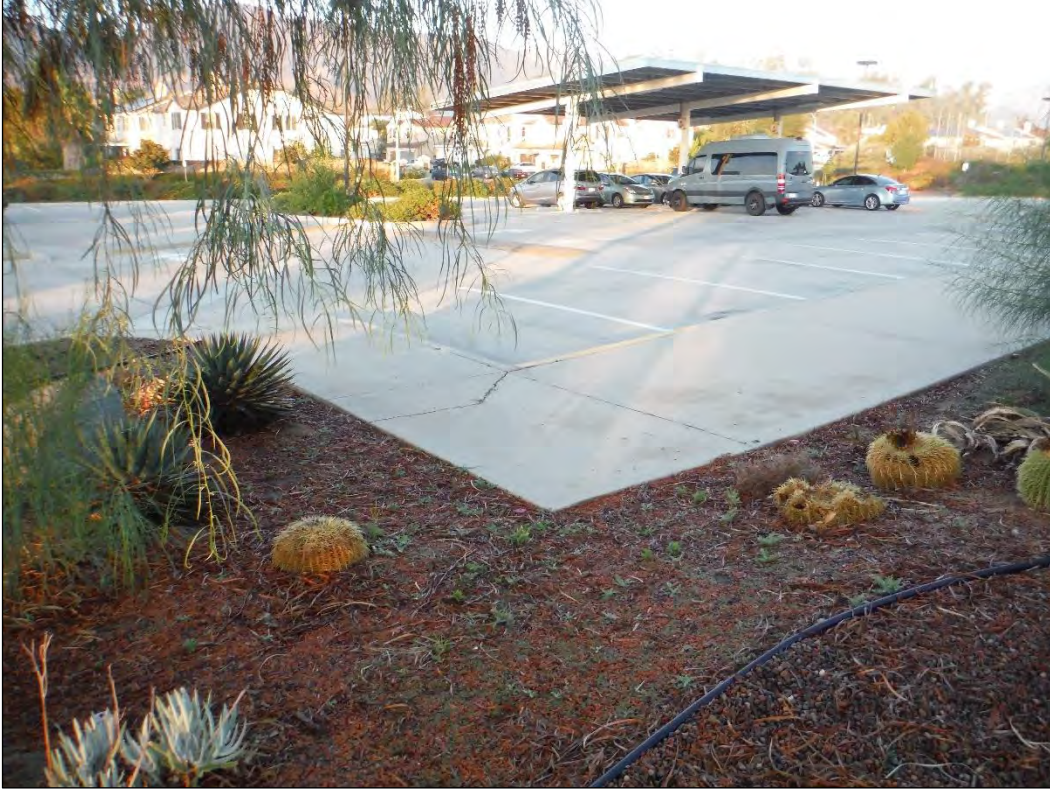
Project overview west, parking lot and landscaping.
